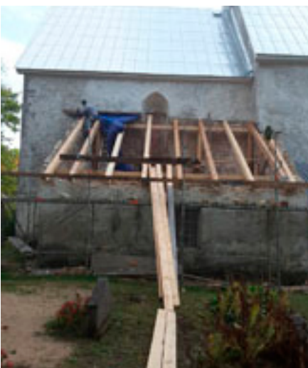
New roof beams in the vestry
