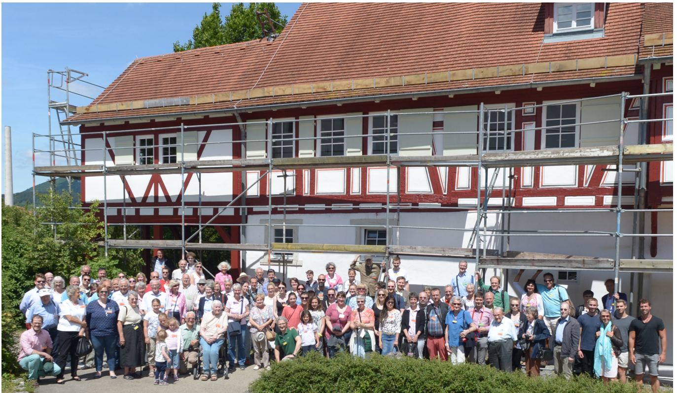
The participants of the family reunion in front of the "Schilling Schlössle" which is undergoing renovation
