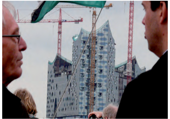
View of the as yet unfinished „Elbphilharmonie“
