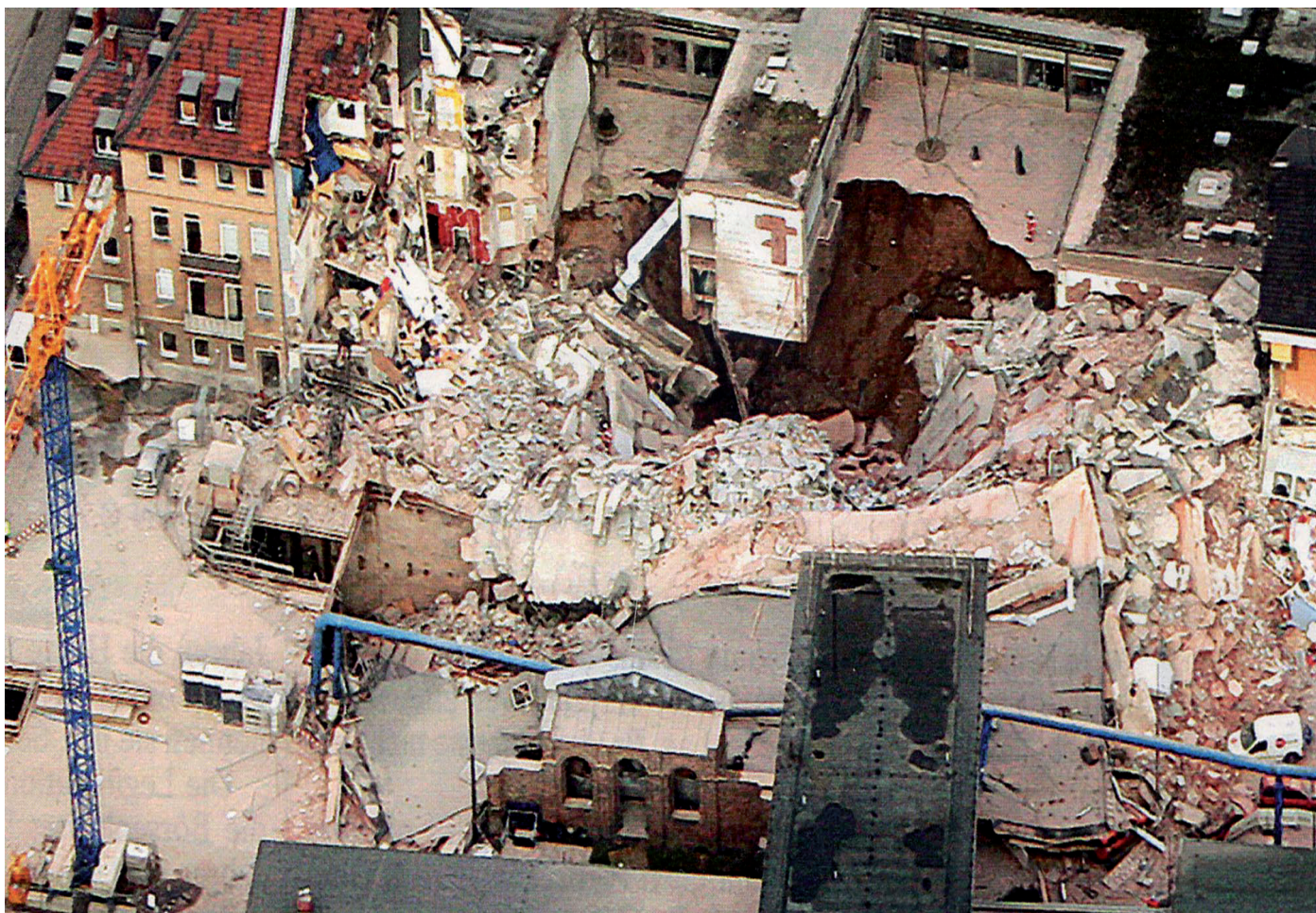
The building of the Historical Archive of Cologne collapsed like a house of cards
