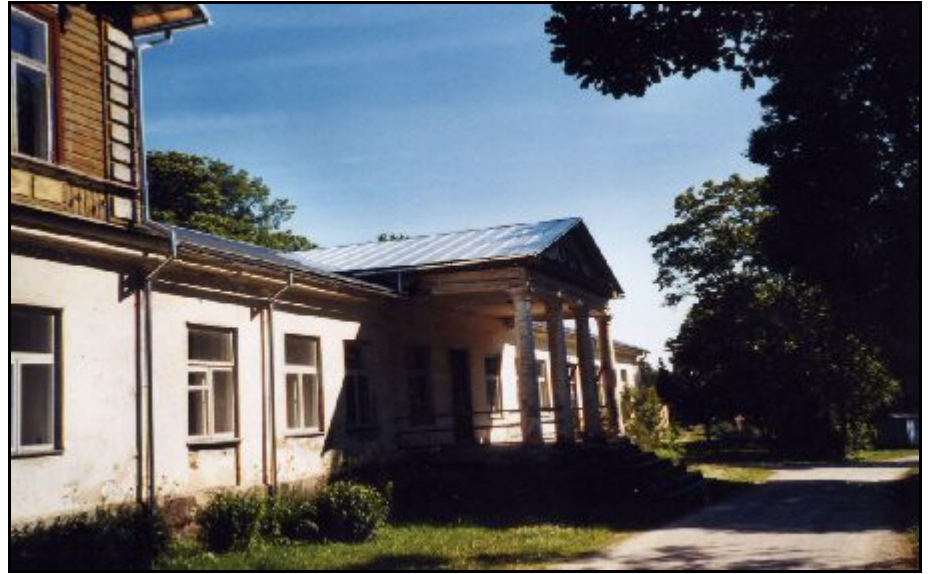
Orgena under new roof
